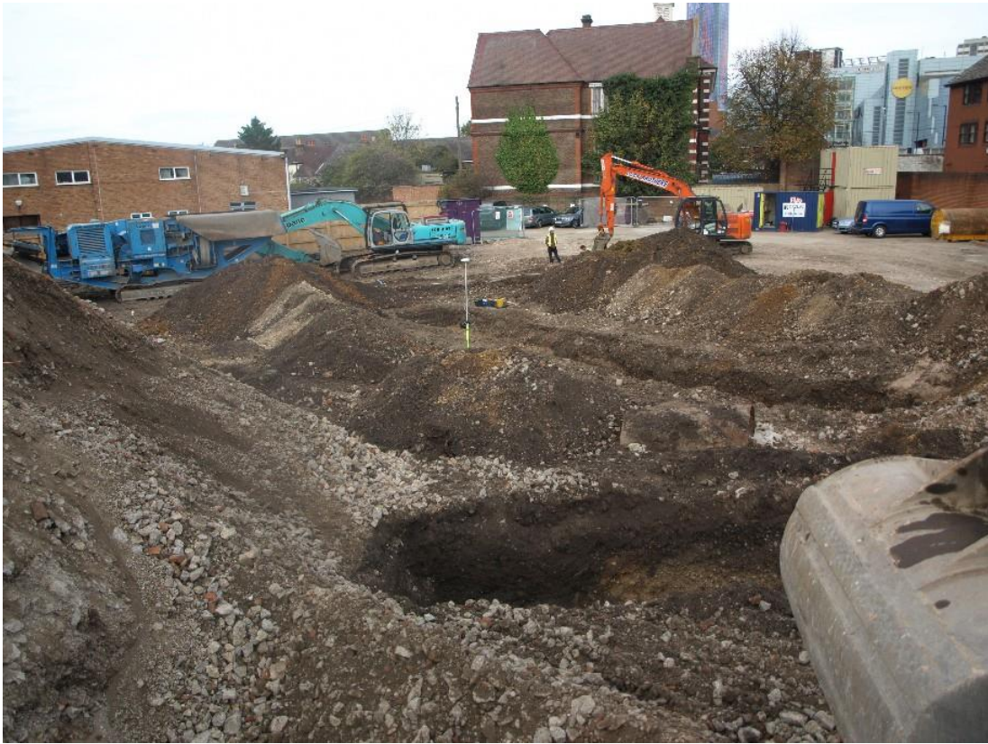
Plate 1: Looking NNE at the site
